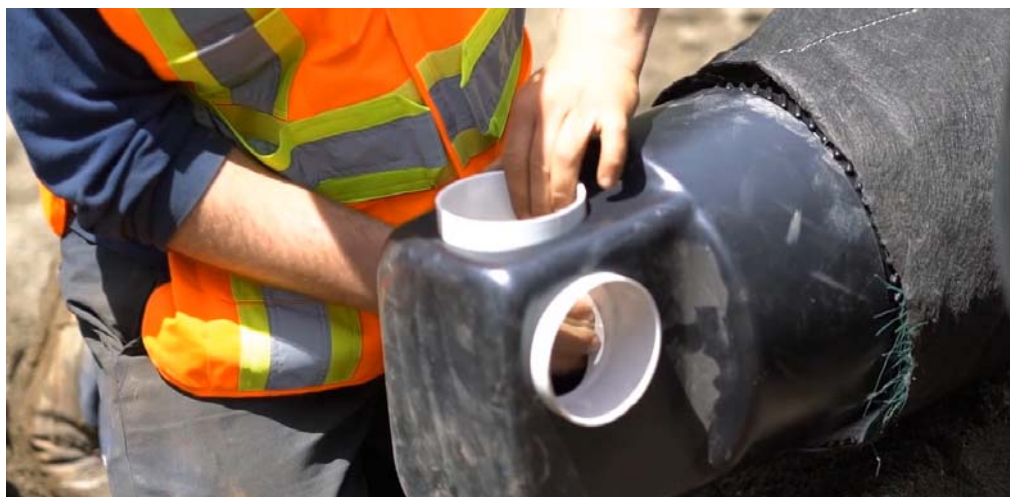
Figure 53. Installation of the piezovent
