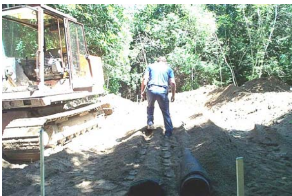
Figure 56. Filling the void around the Advanced Enviro))Septic pipes
