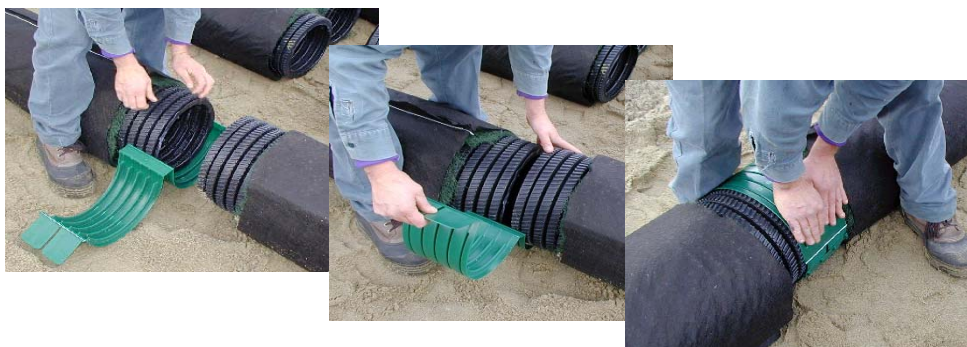
Figure 50. Coupling installation
