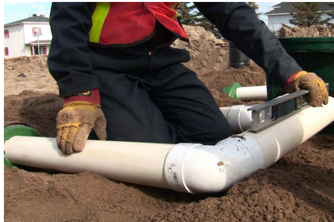
Figure 64. Inlet Pipe sloped toward the System O))
