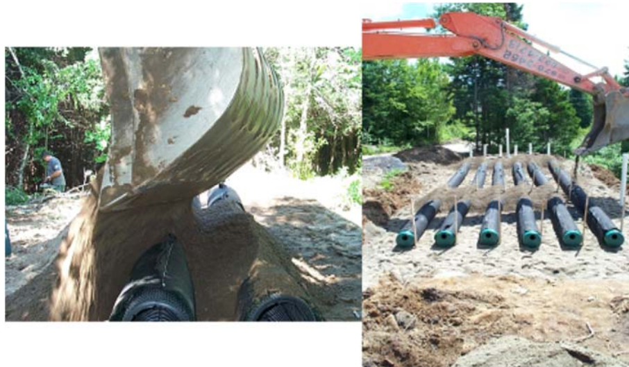
Figure 55. Covering the Advanced Enviro))Septic pipes
