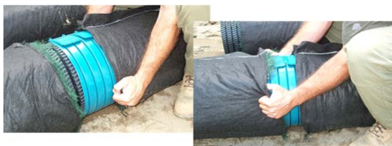
Figure 51. Replacing the membranes over the coupling
