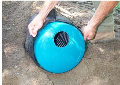
Figure 52. Installation of the Single Offset Adapter
